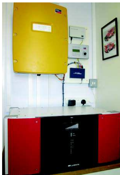
Above SMA’s Sunny Island inverter and Leclanché’s TiBox battery fit snugly into the utility room
